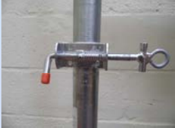
1. SPRING SAFETY LATCH IN THE LOCKED POSITION
