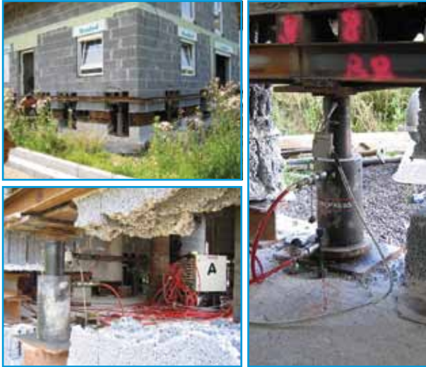
Synchronized lifting with Synchronlift for the rebuilding of house foundations. (Germany 2003)
