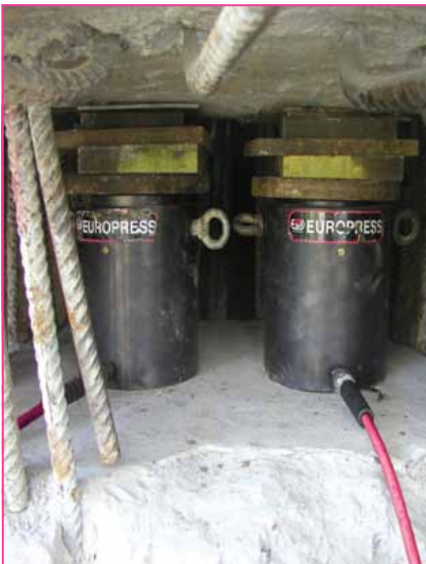
Construction of the "Second Bridge over the Panama Canal - Republic of Panama" for which EURO PRESS has supplied the hydraulic components that hold the segments for the construction of the floor system of the bridge (Panama, July 2003)
