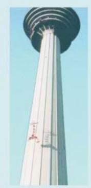
**TIRAK**<sup>®</sup> installed above the load under the upper part of the tower
