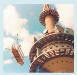
Lifting a component for a **TIRAK®** round platform using a return pulley block system.
