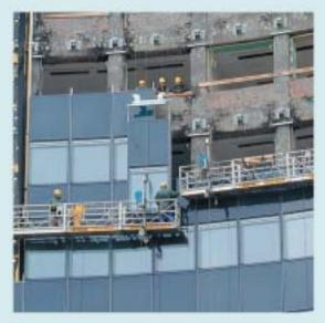
Facade assembly with lifting work platforms. Facade units are moved to the required position in the same way, using  $\textbf{TIRAK}^{\circledast}$  hoists.
