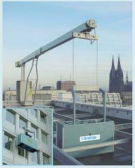
Facade inspection installation with moving trolley on roof – the **TIRAK**<sup>®</sup> is installed on the centralised control platform.
